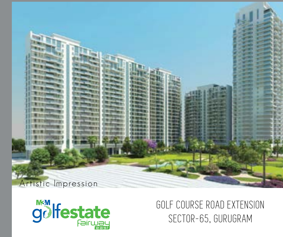
Artistic Impression M3M Golfestate Fairway East GOLF COURSE ROAD EXTENSION SECTOR-65, GURUGRAM
